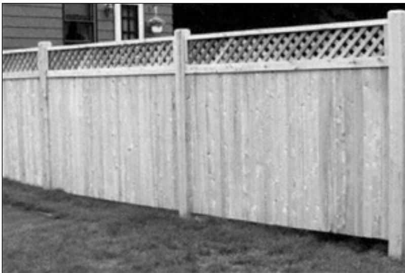
Figure A1-4: Six foot privacy fence, vertical board with one foot of lattice.
